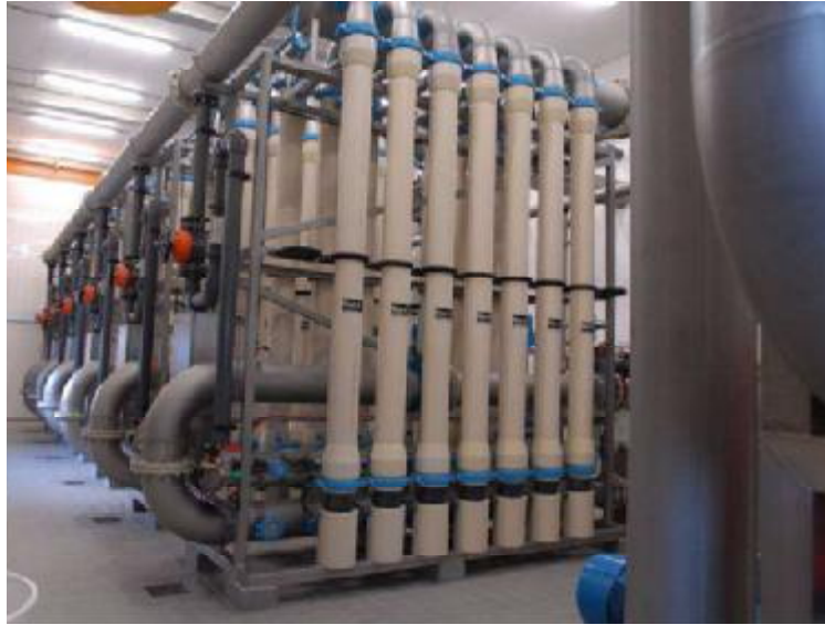
Figure 9: vertical aerated cross flow tubular membranes (origin: Norit X-Flow BV, WEHRLE Umwelt GmbH)
