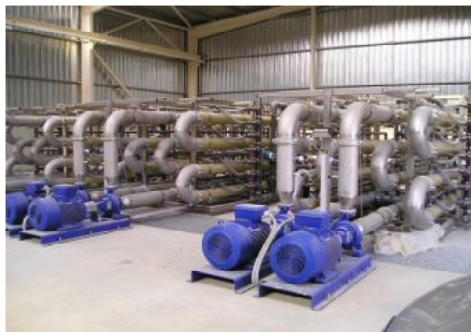
Figure 8: MBR with horizontal cross flow tubular membranes (origin: Berghof Filtrations- und Anlagentechnik GmbH & Co KG)
